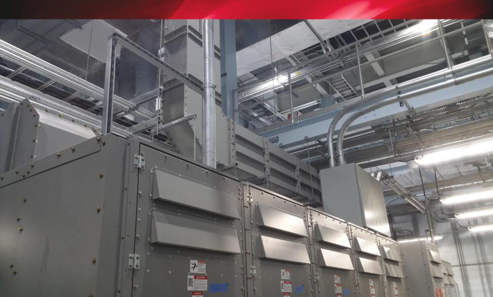
Typical mechanically-vented arc resistant switchgear exhaust plenum area
